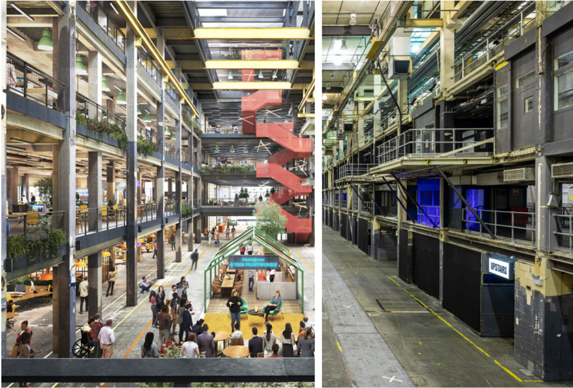
Image: existing internal layout on the right and proposed illustrative view post conversion on the left
